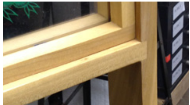
Detail image of a dado joint on the large frame.
