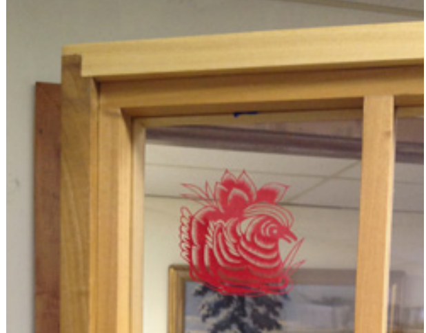
Detail image of the a rabbit joint on the corner of the large frame.
