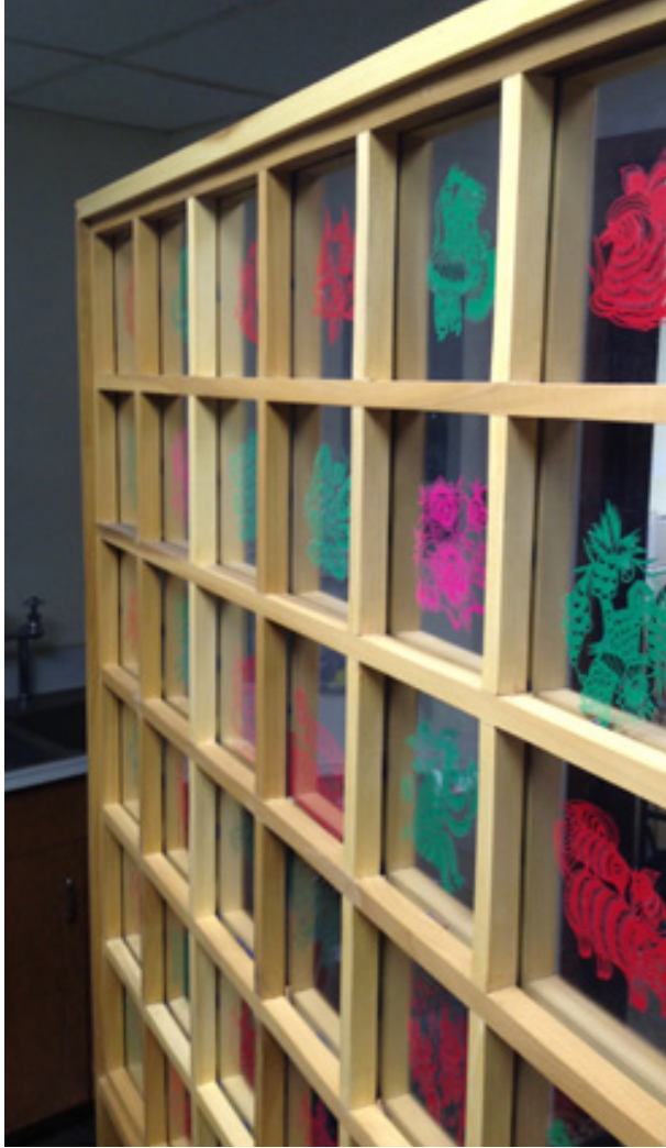
Above: image of the large frame displaying the half-lapped lattice work that secures the plexi-glass.
